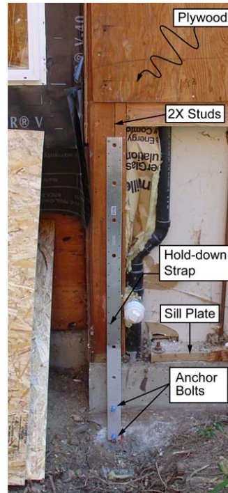
Figure 4b: Hold-down repair installed
