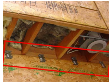
Figure 8: Installation of shear transfer clips
